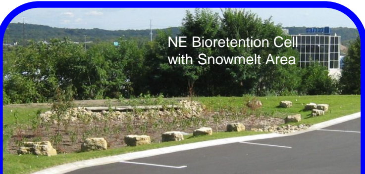
The NE and SE cells have a 3 foot depth of sand/compost media and 6" subdrains to provide biofiltration treatment. Temporary pool depths are limited to 12 inches maximum.
