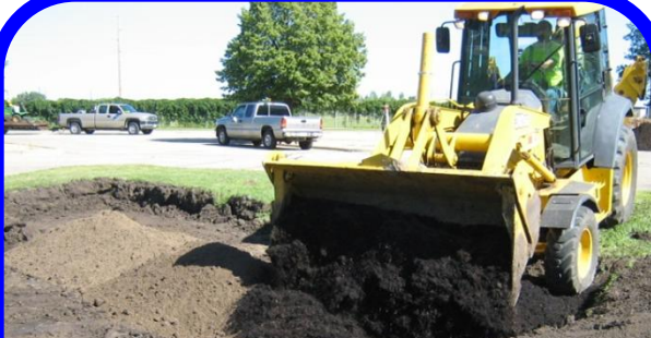
In existing soil was amended with coarse washed sand and leaf litter compost. Mixing to a 12" depth helped to remove soil compaction.
