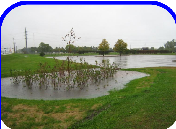
The designed water quality volume of \frac{1}{2} inch runoff depth fills the cells to capacity. The temporary pool infiltrates within 12 hours following the rain event.
