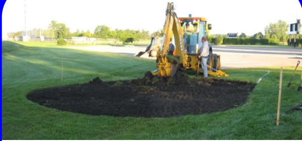
Existing utilities were located before removing turf layer.
