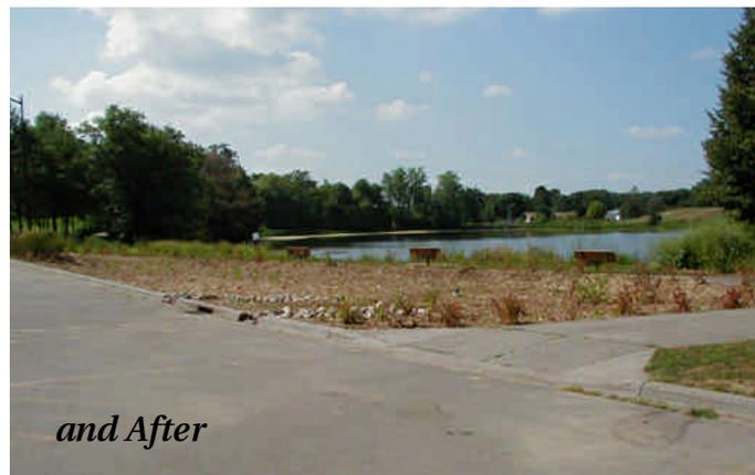
water garden design incorporated soil corrections, an underdrain system, curb cuts to allow water to flow into the rainwater garden, and native plantings. The rainwater garden area is roughly three thousand square feet and obtains a water ponding depth of eight inches. Total storage is estimated at fifteen thousand gallons prior to overflow through an emergency outlet.
