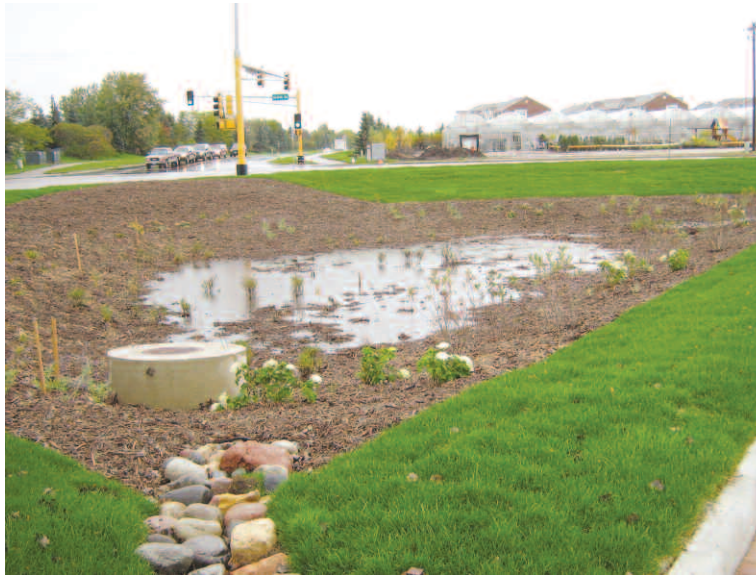
Newly installed raingardens capture runoff from the parking lot
