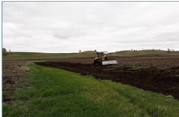
The waterway was graded to meet the new design.
