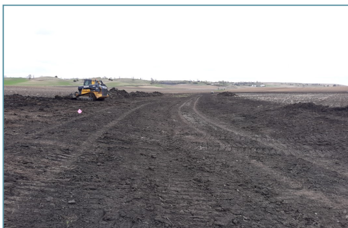
Salvaged topsoil was respread after grading of the waterway.
