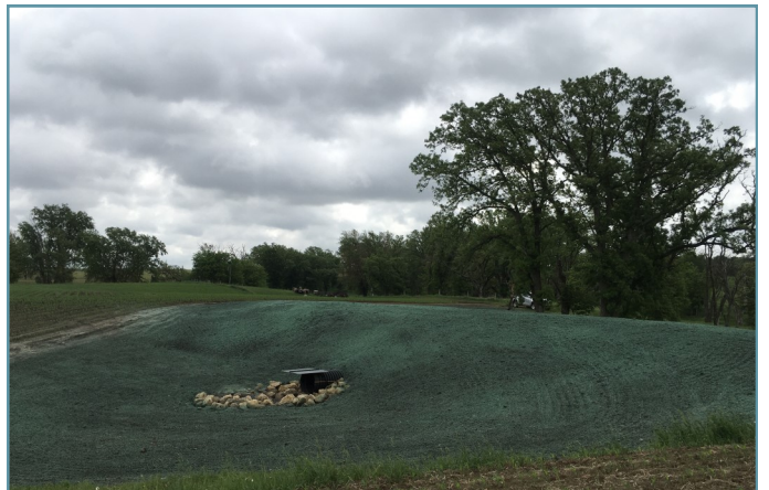
The finished embankment was seeded with perennial vegetation and hydro-mulched.
