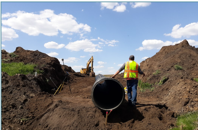
A new HDPE pipe was installed.
