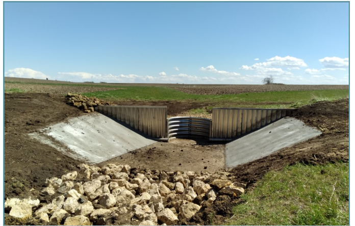
View of completed project
