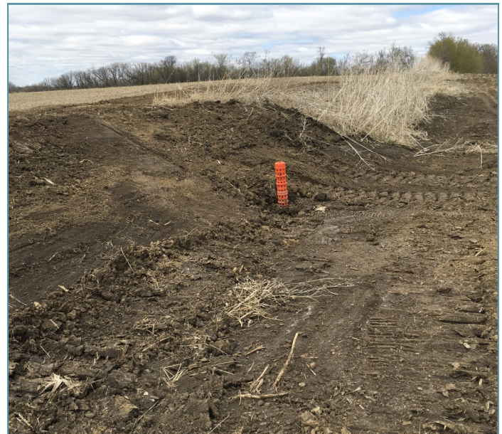
Photo of the repaired project
