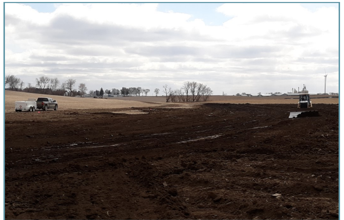
The waterway was graded to convey surface water runoff.
