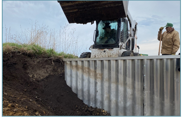
Eroded areas around the wing wall were repaired.
