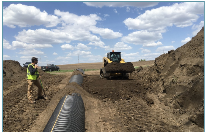
The embankment beside and above the pipe was reconstructed.
