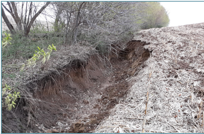
Gully erosion was occurring along the property edge.
