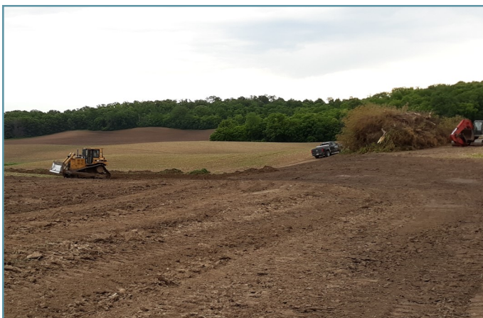
The grassed waterway and critical area planting were graded.
