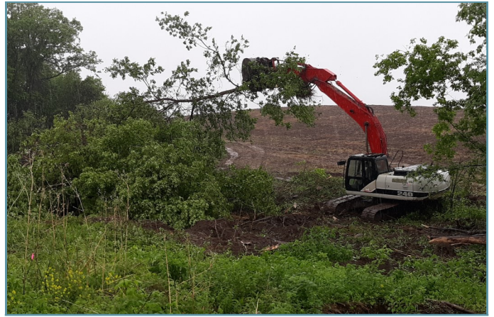
Trees were cleared throughout the project area.
