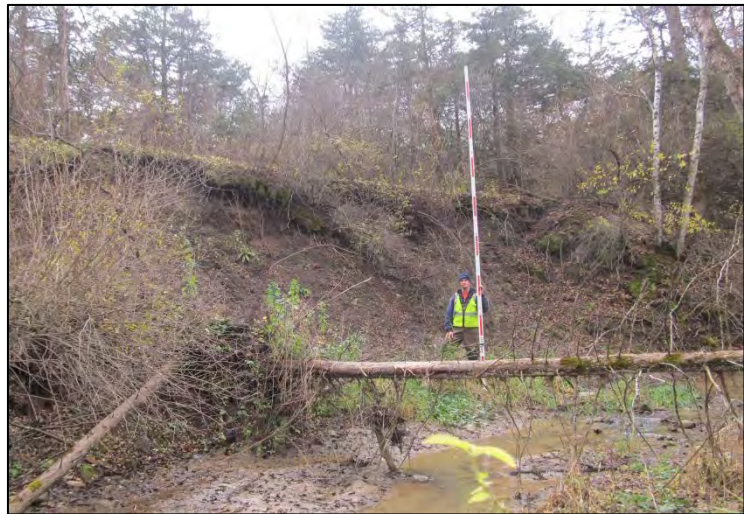
Example of location identified for streambank stabilization
