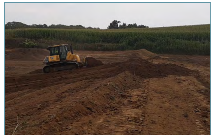
Berms were constructed for each basin and finished with topsoil.
