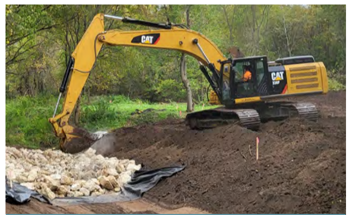
Rip-rap ditch checks were installed to prevent future erosion.
