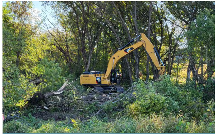
Fallen trees were cleared at the beginning of construction.
