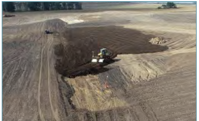
Topsoil was spread over each of the farmable basins after construction.
