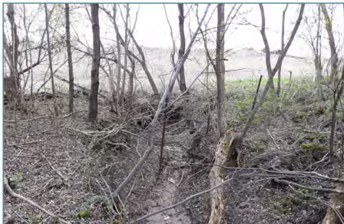
A gully had formed through the trees near the fence line.
