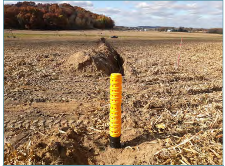
A riser inlet will control the release of water from the basin.
