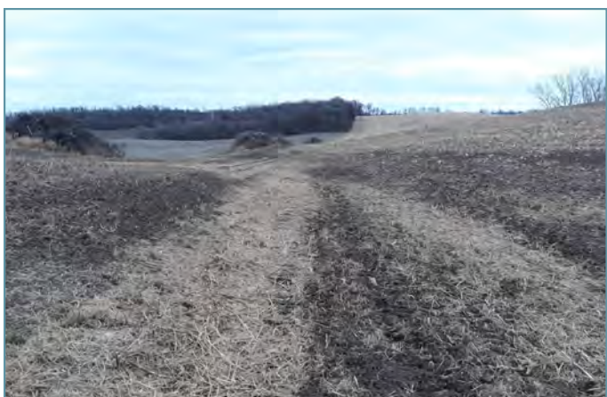
The waterway was seeded and mulched.
