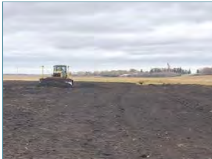
The waterway was graded using a dozer.
