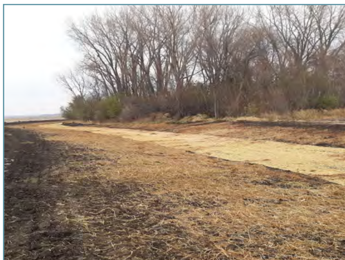
Straw mulch was broadcast and anchored to further reduce erosion.
