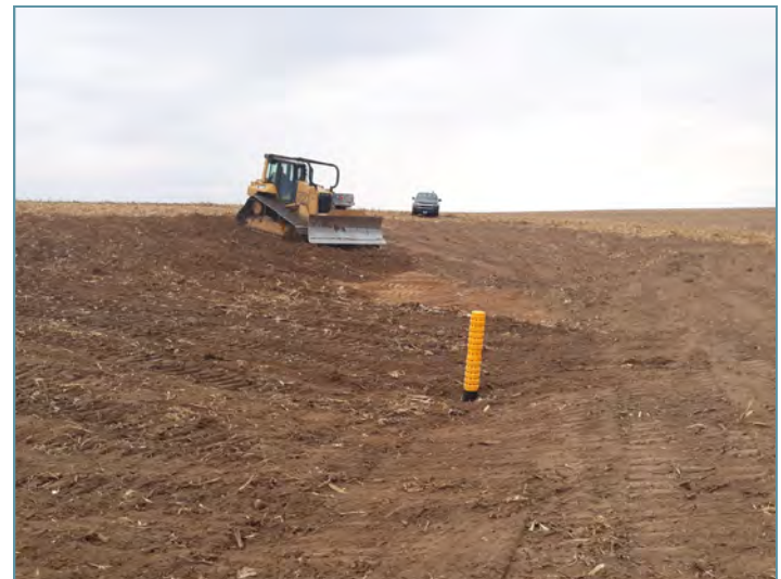
A berm was constructed and basin grading was completed.
