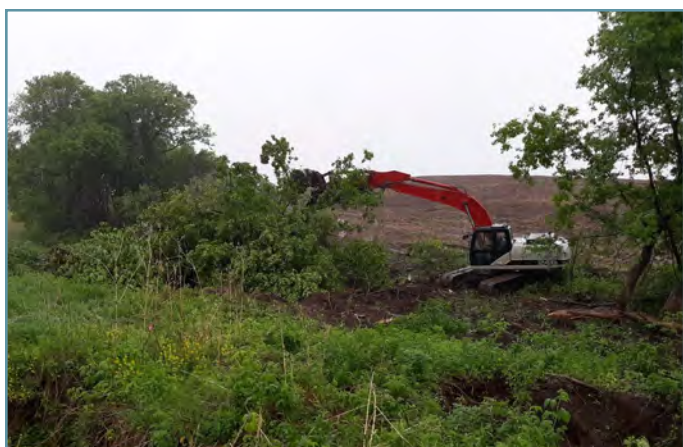
Trees were removed to allow for grading.
