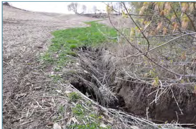
The existing gully was actively eroding.
