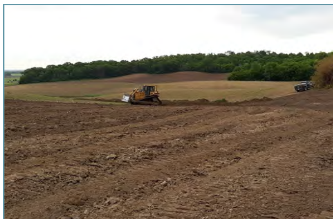
The waterway and hillside were graded.
