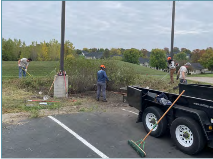
Crews clear vegetation from the Hastings Corrections facility rain garden in preparation for new plantings and mulch to be installed.
