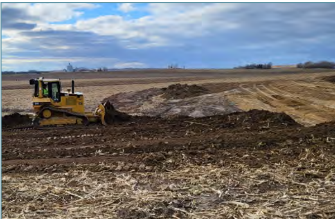
Topsoil was spread over each basin after grading.
