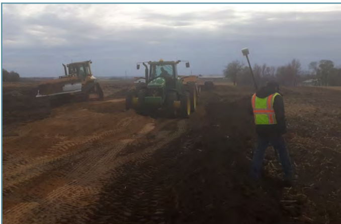
Basins were shaped using scrapers.
