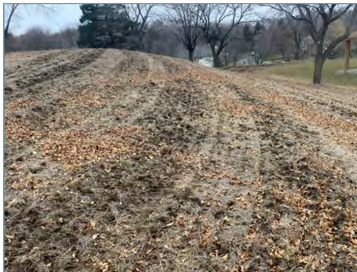
No-till drill seeding occurred across sloped areas to reduce erosion. Seed will germinate in the spring and it will take several years for the prairie to mature.
