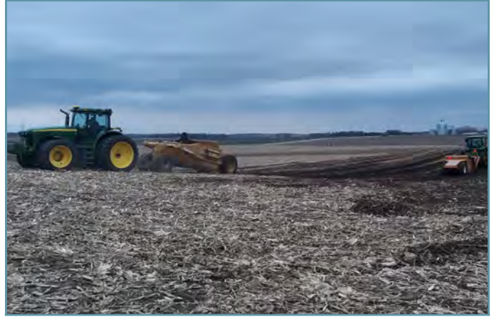
Topsoil was removed and stockpiled using scrapers.
