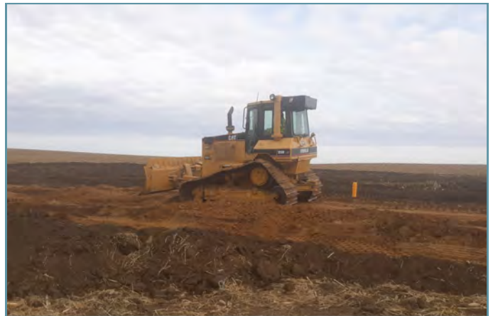
Embankment material was placed and compacted with a dozer.
