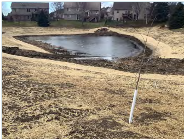
All areas that did not have erosion control blanket were straw mulched to hold seed and soil in place. The straw mulch and blanket will reduce erosion until the native vegetation is established.
