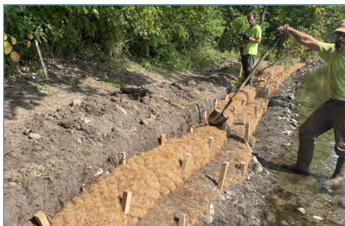
Double stacked coir logs were used in areas with higher banks or where there was heavier foot traffic.
