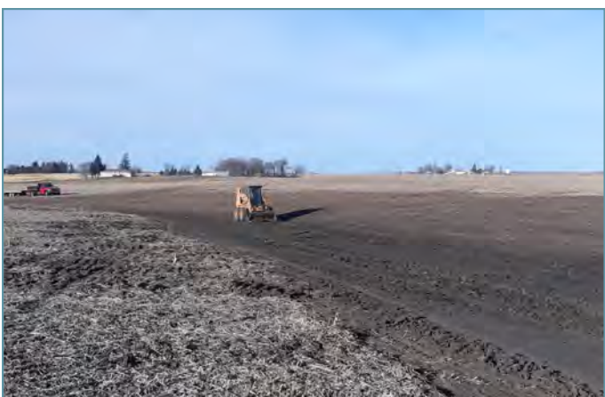
After grading using a bulldozer, the waterway was prepared for seeding.
