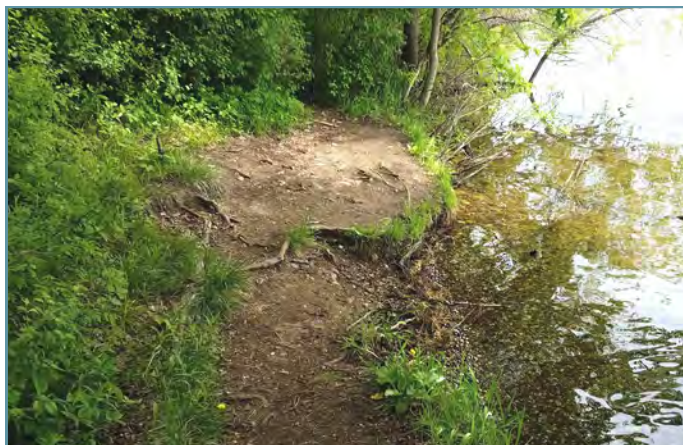
Before the project, heavy foot traffic had smothered vegetation, resulting in erosion and undercut banks.
