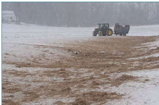
Straw mulch was used to reduce erosion until vegetation establishes in the spring.
