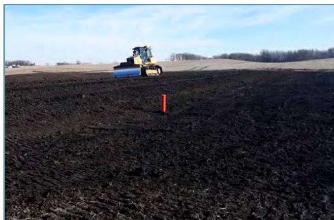
Topsoil was re-spread after the embankment and basin construction.
