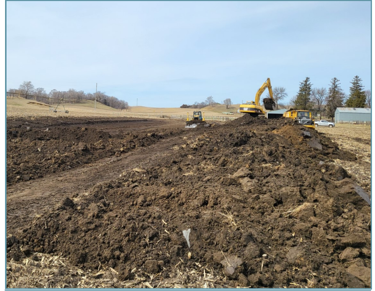
Grassed waterways were graded and shaped to adequately convey runoff.
