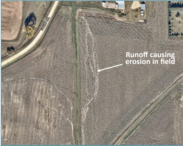
Existing grassed waterways were past their designed lifespan and surface water runoff was flowing alongside the waterway and causing erosion in the field.
