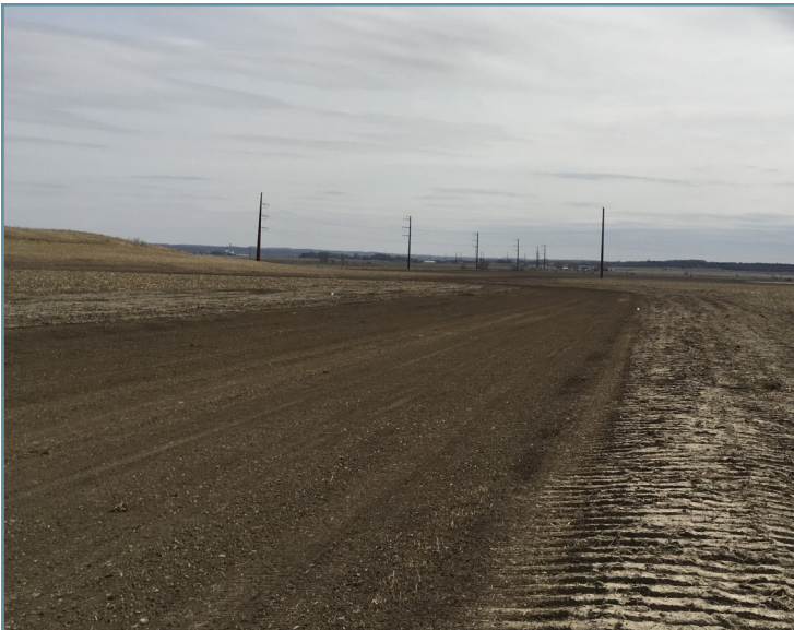
After grading, the waterway was prepared for seeding.
