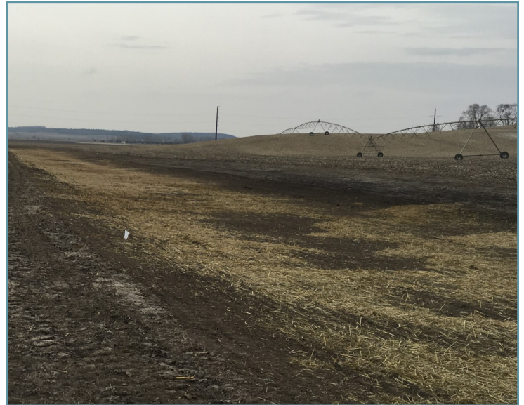
The grassed waterway was seeded with perennial vegetation. Straw mulch was used to reduce erosion until vegetation is established.
