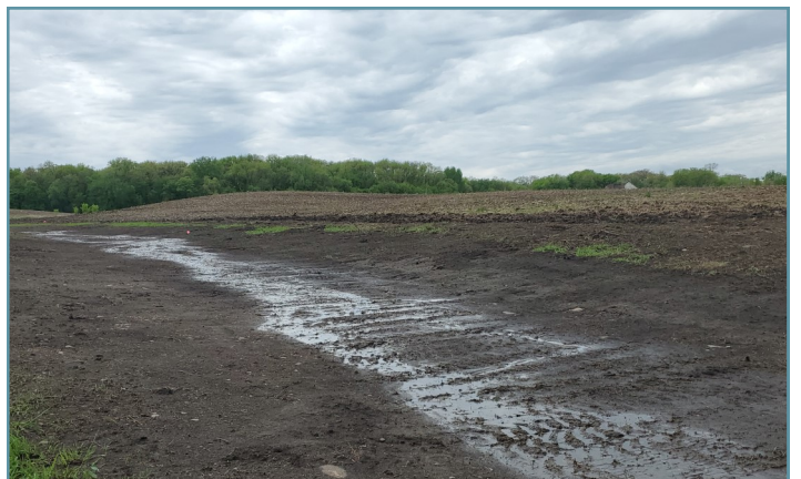
Waterways were graded and shaped to adequately convey runoff.
