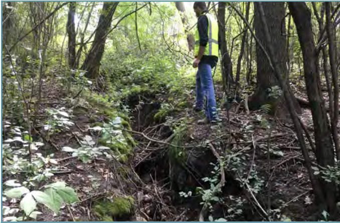
Surface water runoff on a wooded slope caused a gully to form.
