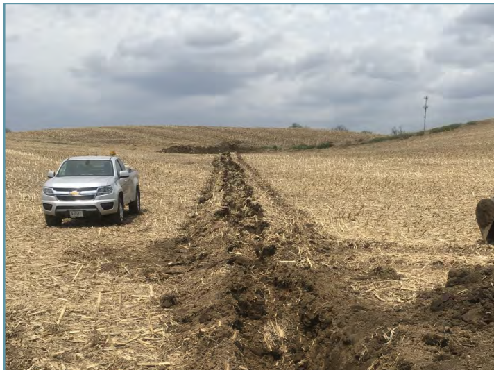
Underground outlet tiles were installed for each basin.
