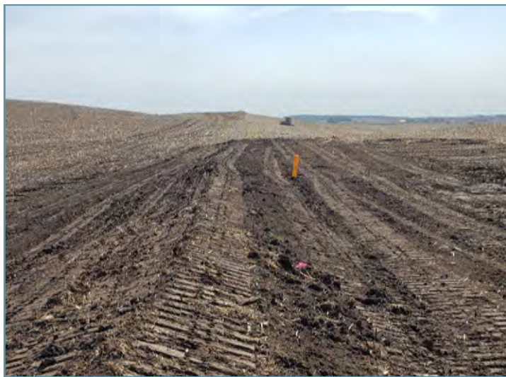
Basins were graded and seeded with a perennial grass mixture.
