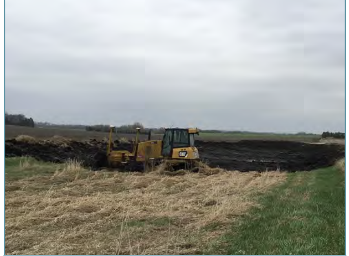
1,500 feet of grassed waterway was graded.
