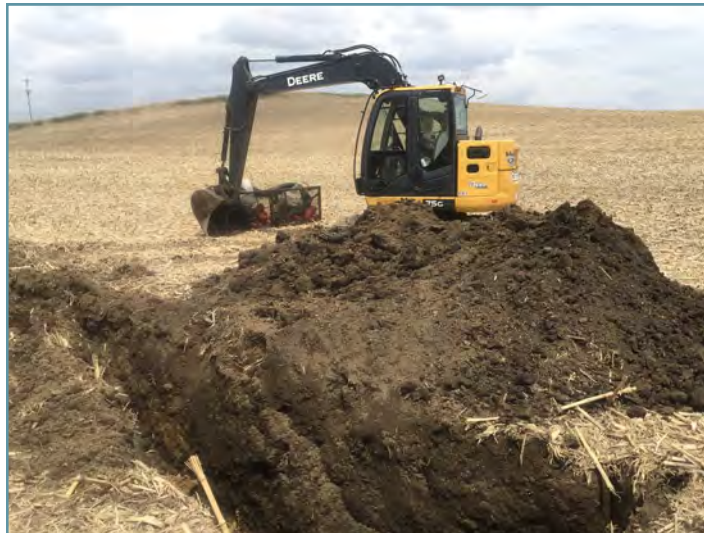
Basin inlet structures were installed.
