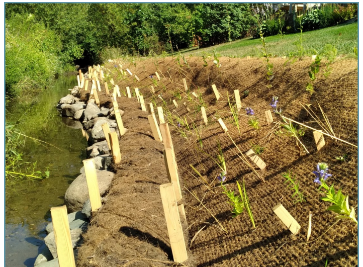
The completed project will reduce future erosion and provide pollinator habitat.
