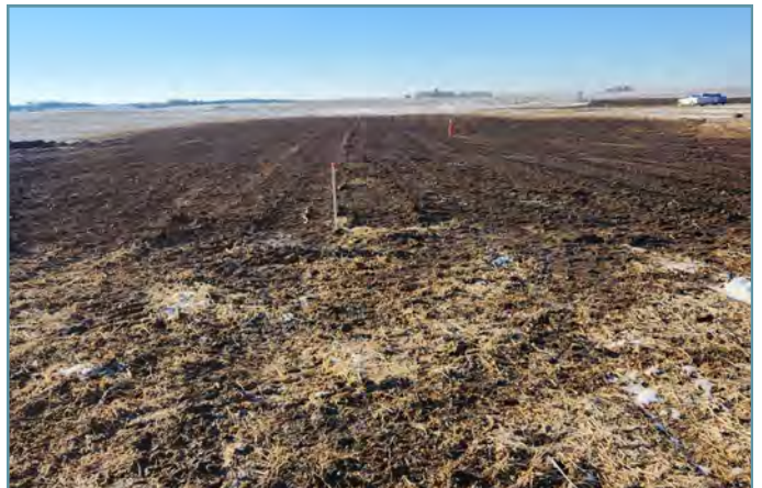
The second basin has embankment slopes that are flat enough to be farmable.
