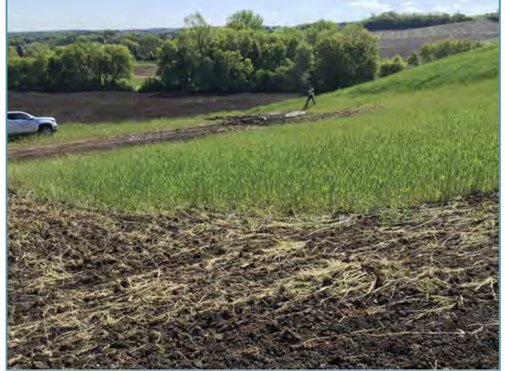
The project area was surveyed and a water and sediment control basin was designed to capture runoff and slowly release it through an underground outlet.
