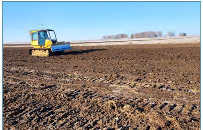
After shaping, topsoil was spread throughout the area.
