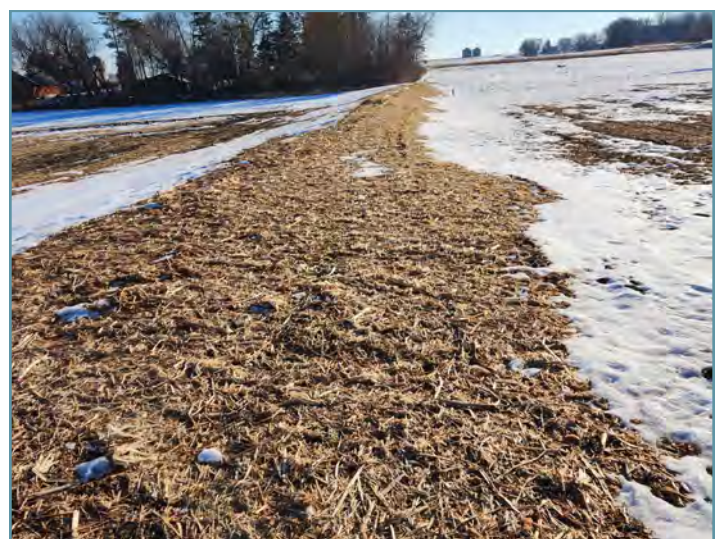
The embankments on each of the water and sediment control basins were seeded with perennial vegetation and mulched.
