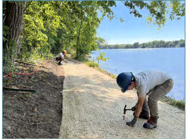
The old trail area was re-graded, with topsoil for plant growth, seed and erosion control blanket was installed with wooden biodegradable stakes, and finally plant plugs throughout.
