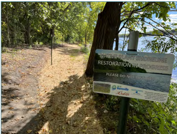
Signage indicates the intent of the project and asks users to stay off. Temporary fencing (installed later on stakes) further helps keep foot traffic off until new plants establish.
