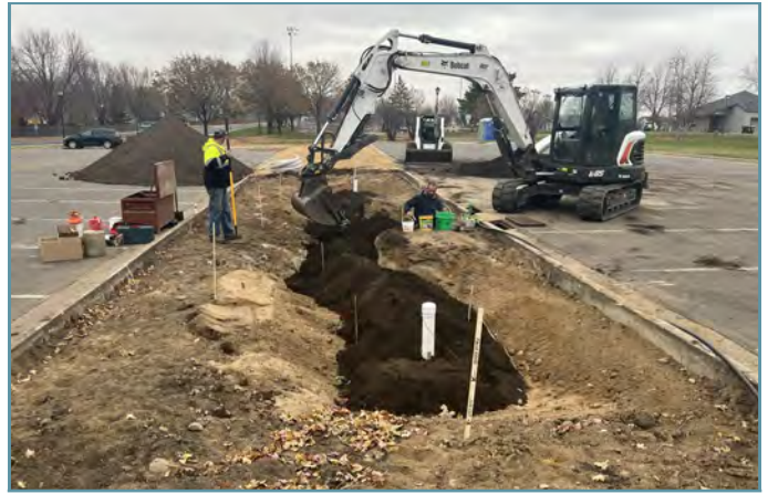
A sand and compost soil mix was added to the basin. The soil mixture is permeable and supports plant growth.
