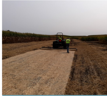
Constructed 4,860 linear feet of grassed waterways
