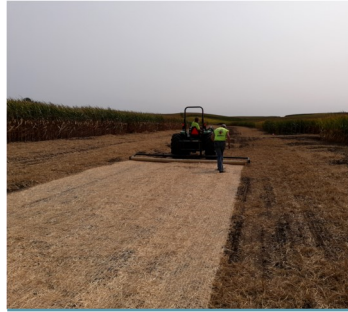
Constructed 4,860 linear feet of grassed waterways
