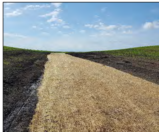
Example of a recently constructed a grassed waterway within the Mud Creek subwatershed
