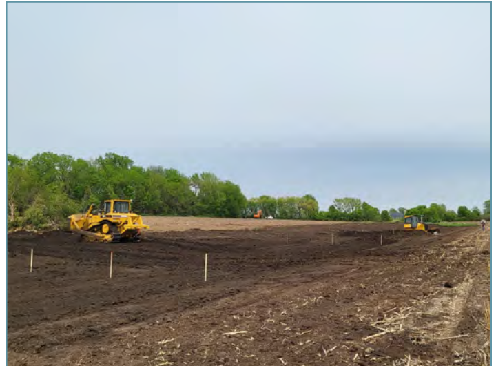
Accumulated sediment was removed and the grassed waterways were reshaped.
