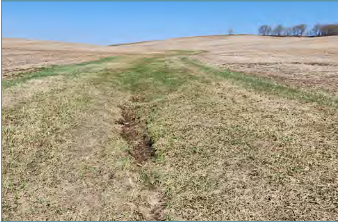
Concentrated flow was causing erosion in the existing waterway channel.
