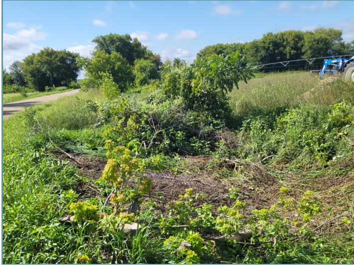
Trees were removed from the construction area.
