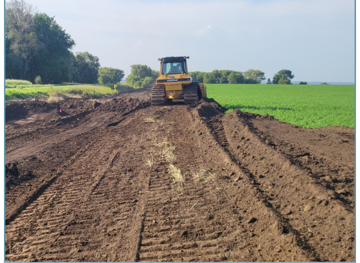
The new waterway was shaped to adequately convey surface water runoff.
