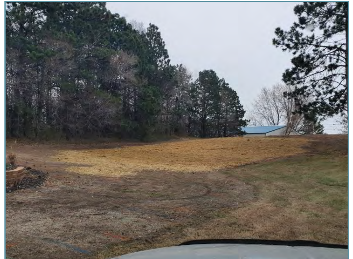
Following seeding, mulch was applied to prevent erosion.
