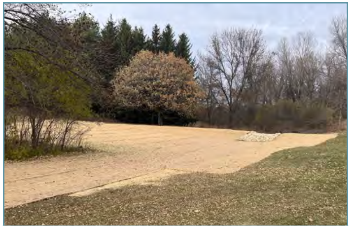
The basin was seeded with native vegetation and erosion blanket installed.
