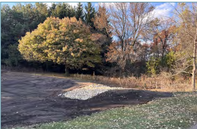
Topsoil was placed and an emergency spillway was constructed using rock.
