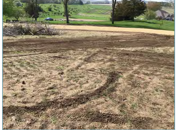
Turf grass areas were treated with herbicide to remove existing vegetation.
