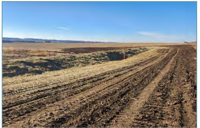
The completed basin will slow runoff and reduce future erosion.
