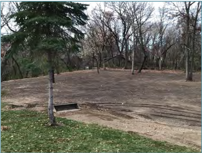
Following tree and vegetation removal, soil was prepared for seeding.
