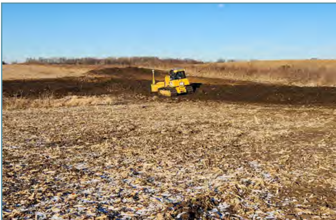
Topsoil was stripped and stockpiled to use after grading.
