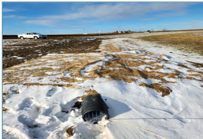
Runoff is released through a tile that outlets to a recently constructed grassed waterway.
