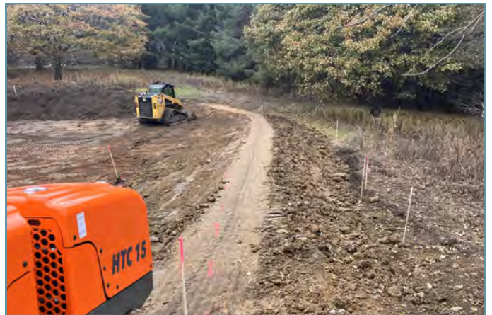
The embankment was compacted to ensure it holds back water.
