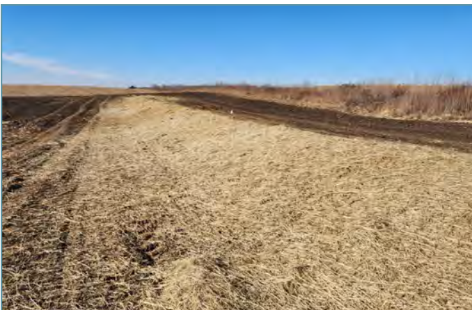
Seeding and mulch was installed to vegetate and stabilize embankment.
