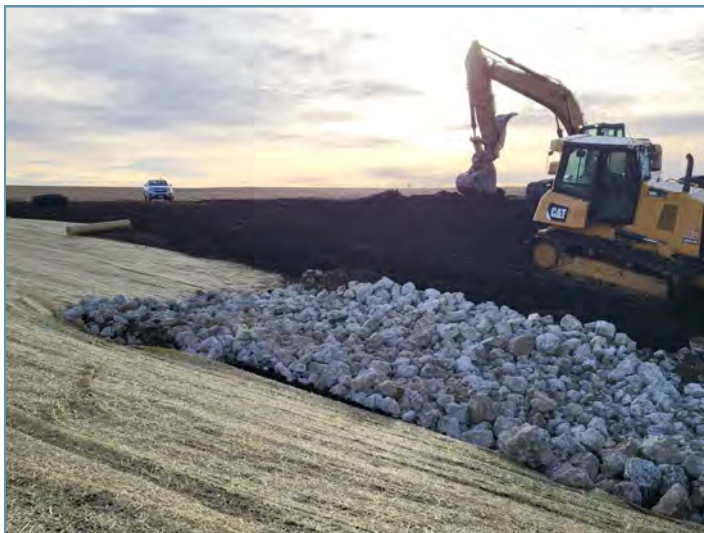
A rock lined waterway was constructed to protect soils where runoff had the greatest potential to cause erosion.
