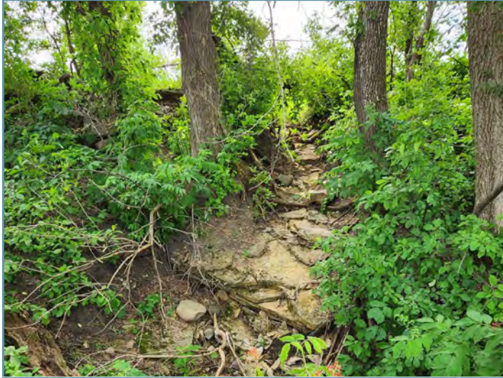
Concentrated runoff was causing gully erosion.
