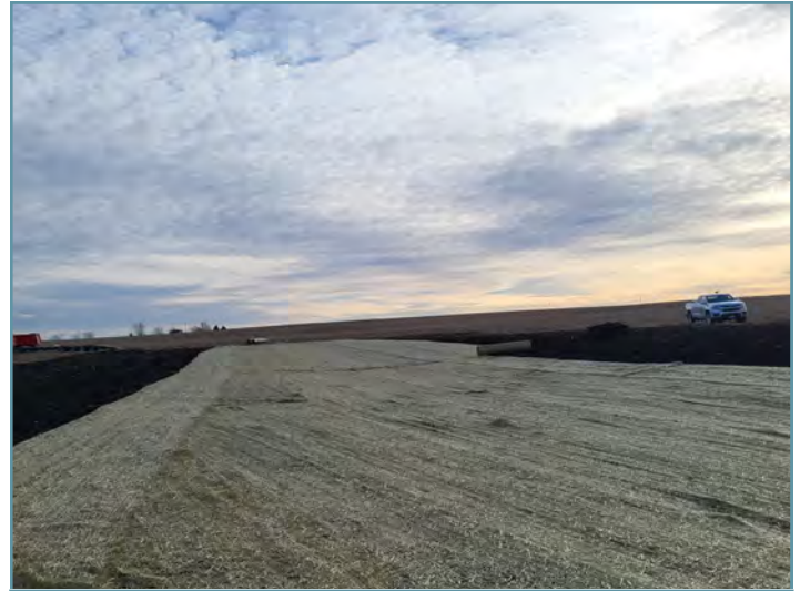
A 200 foot grassed waterway was constructed.
