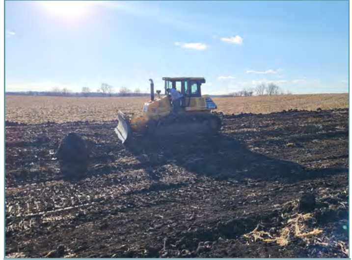
Topsoil was stripped in preparation for grassed waterway construction.
