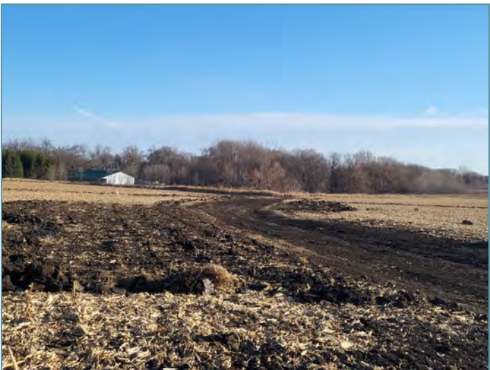
The grassed waterway was graded to convey runoff.
