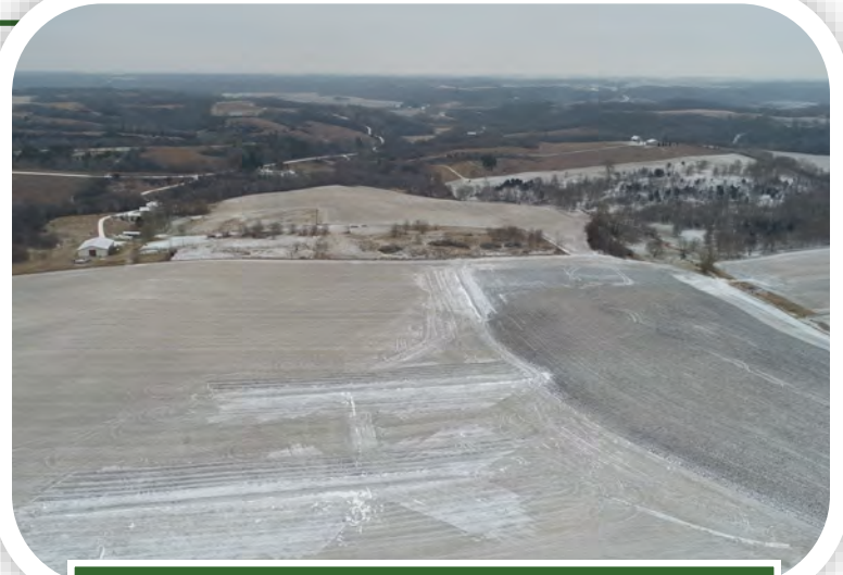
A series of three basins installed to reduce soil erosion in the Little Cannon River Watershed in Goodhue County
