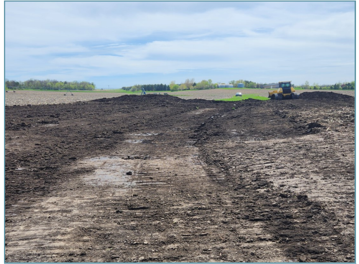
A dozer was used to shape the waterway.
