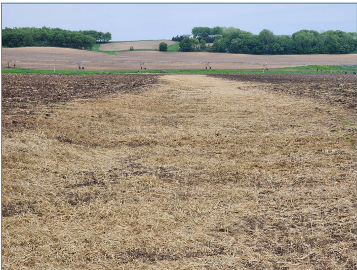
After replacement of topsoil, the waterway was seeded with perennial grasses and mulched to reduce erosion.
