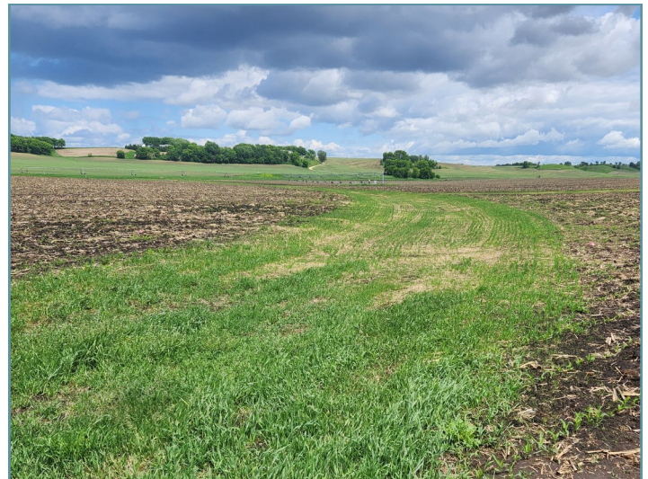
The reconstructed waterway will convey runoff and reduce future erosion.
