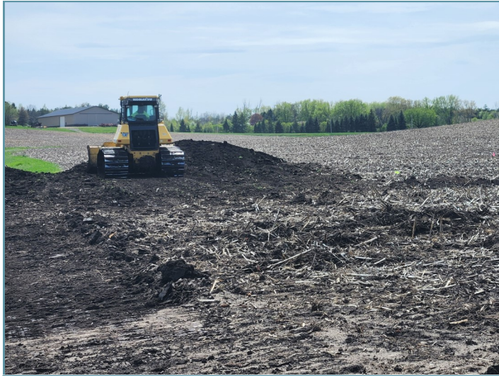
Topsoil was cleared from the project area and stockpiled.
