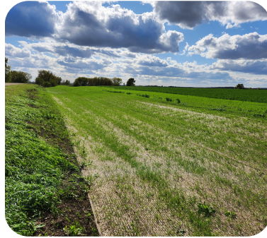
Constructed 8,257 linear feet of grassed waterways
