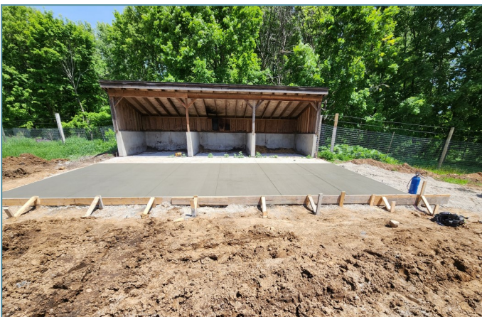
Concrete pad was allowed to cure before removing forms.
