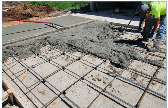
Concrete was poured and reinforced with rebar.
