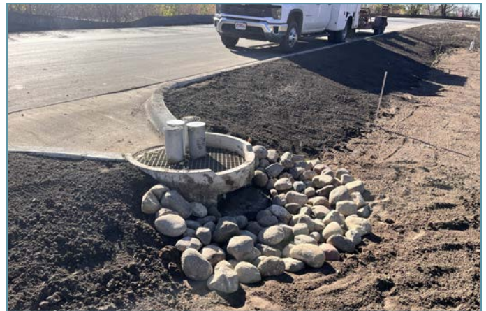
A pre-treatment structure was installed to capture coarse sediment.
