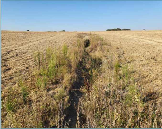
Gully erosion was occurring in two areas of the field prior to the start of construction.
