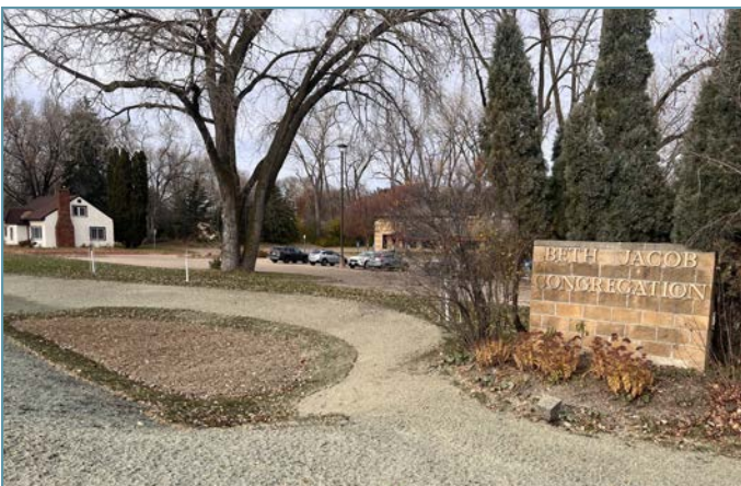
Sod was placed immediately around the basins and hydroseed was placed outside the sod for final stabilization.
