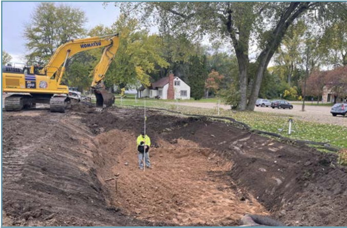
The existing soils were removed down to well-draining subsoils.
