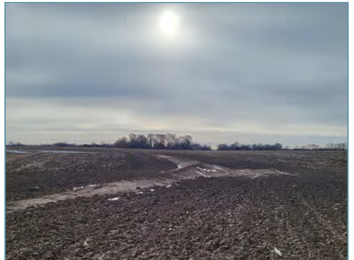
The upper basin was reconstructed and an underground outlet was added to convey runoff and reduce future erosion.
