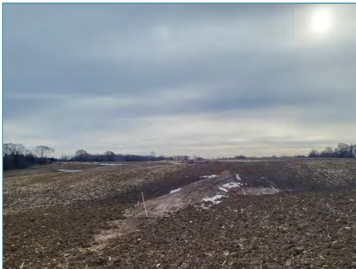
The lower basin was reconstructed to increase holding capacity.
